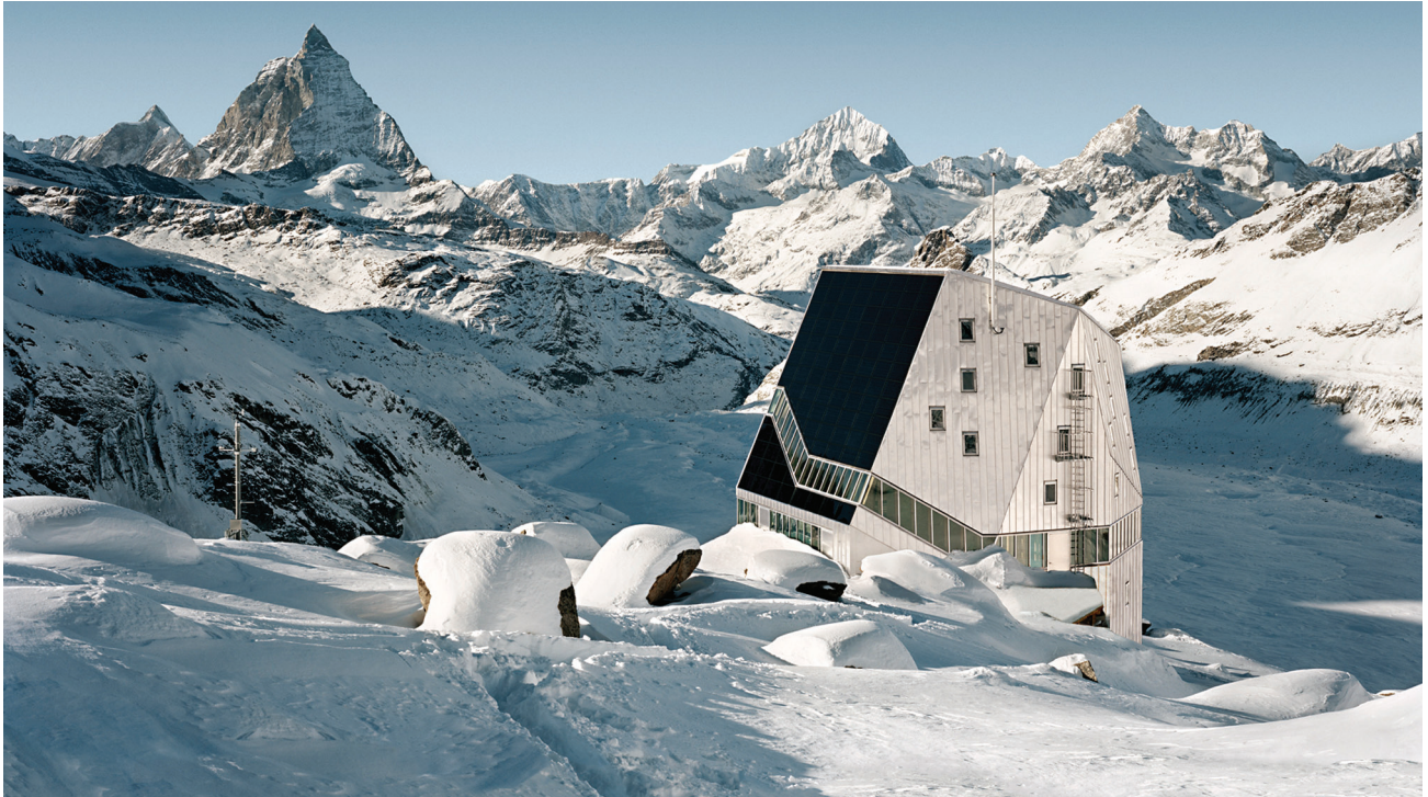
Fig. 5: There are no limits to sustainable building, even in the middle of a glacial landscape. A prime example of this is the “New Monte Rosa Hut Project” (2883 m a.s.l.), a joint venture between ETH Zurich and the Swiss Alpine Club SAC. The new hut was officially opened in autumn 2009 and is designed to achieve a self-sufficiency rate of at least a 90 percent, thus setting a global milestone in energy-efficient building: www.neuemonterosahuette.ch
